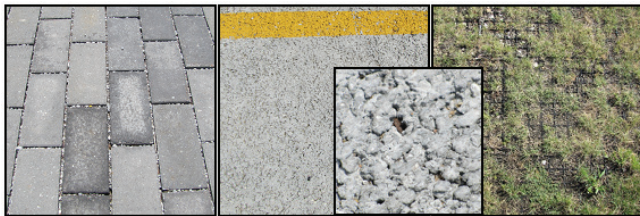
Figure 7. Permeable pavers (left); porous concrete and close-up (center); grass paving grid (right).
