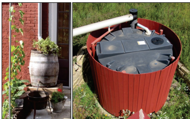
Figure 3. Rain barrel constructed from a repurposed whiskey barrel (left) and a 3,000 gallon cistern (right).
