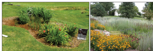
Figure 4. Rain garden (left) and bioretention basin (right).
