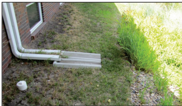
Figure 9. Downspout extensions and splash blocks directing roof runoff to a rain garden.
