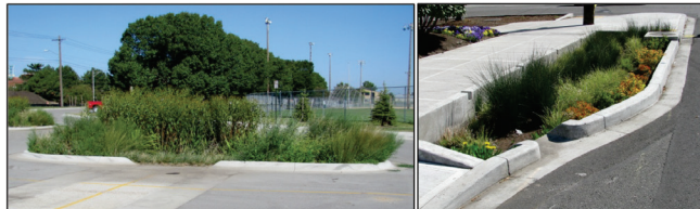
Figure 8. Curb cuts into parking lot island (left) and rain garden in street right-of-way (right).
