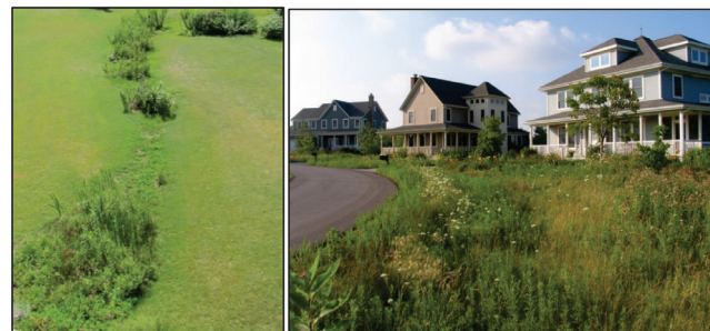
Figure 5. Bioswales. Streetside bioswales (right) can sometimes be used in place of a system of street curbs, gutters, and underground storm drains.
