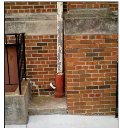
Figure 1. Downspout routed into a sanitary sewer connection – an illegal practice.
