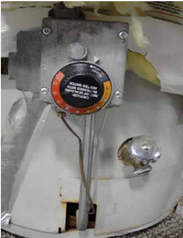
Figure 3. Turn down water heater temperature according to manual.
