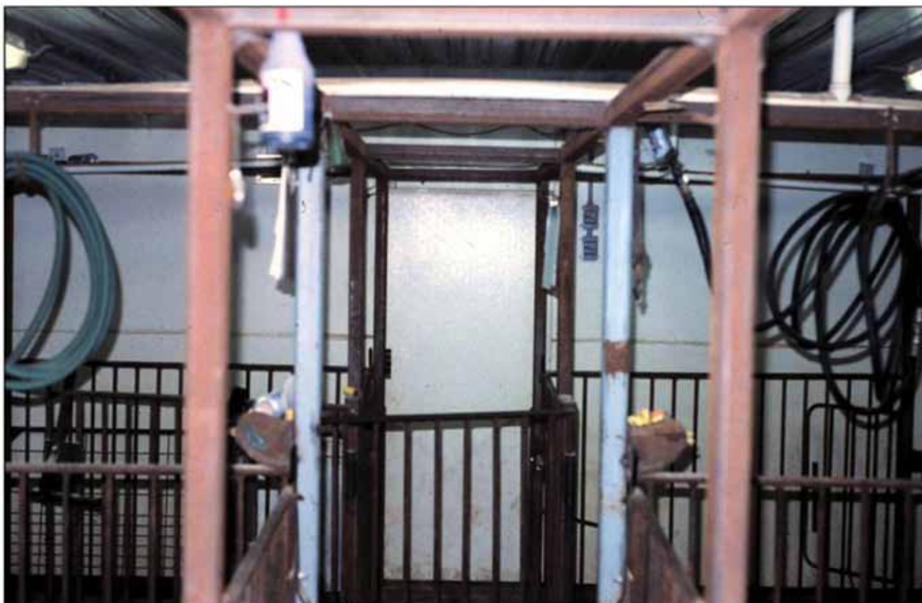
Picture 9. An overhead structure to prevent gate latch corner post from moving.
