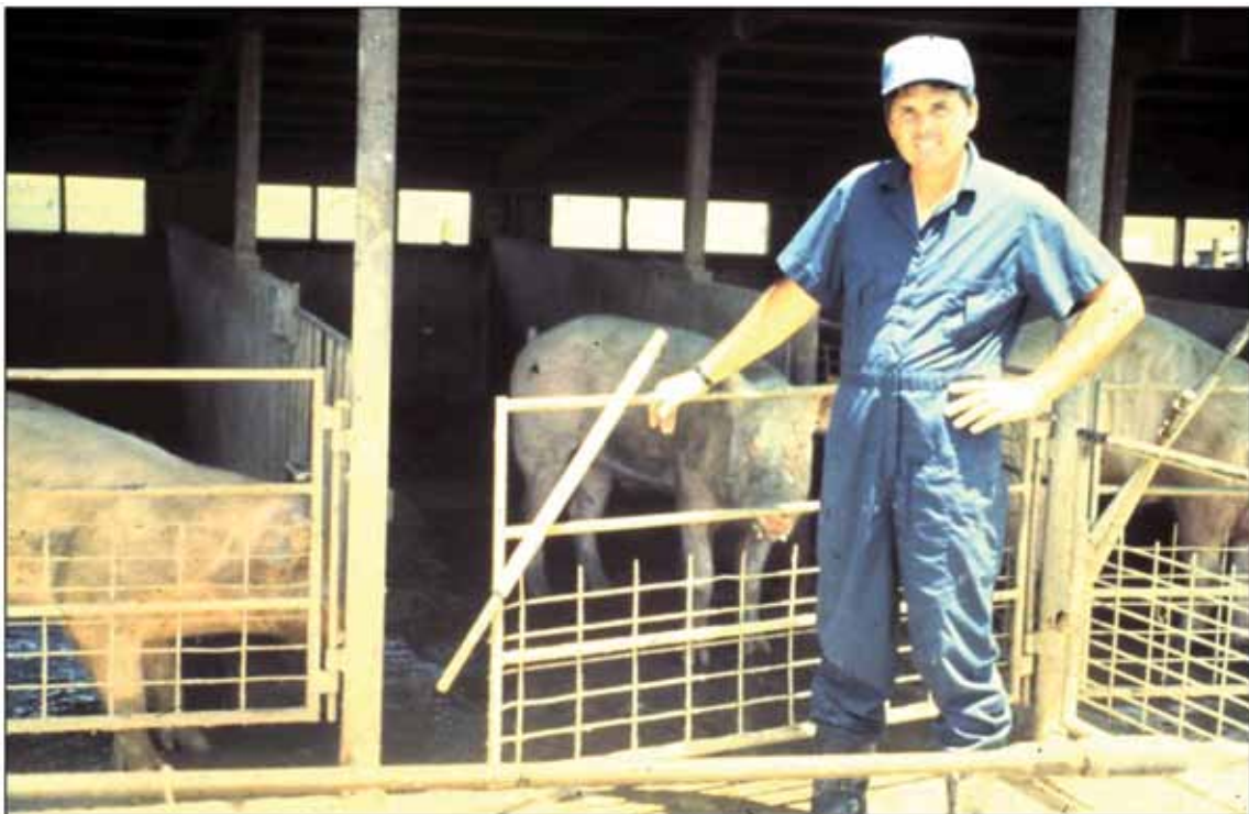
Picture 2. An angle rod slides into a hole in the steel post that supports the roof of the building.
