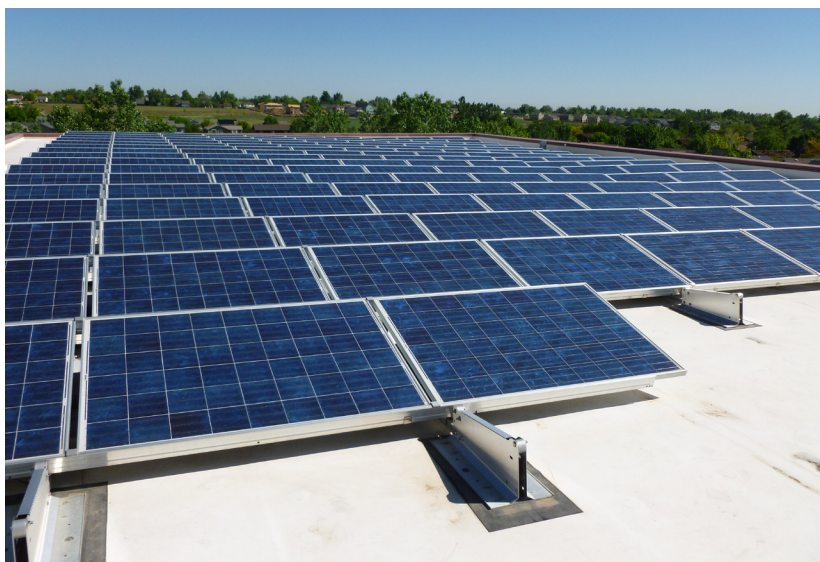
Figure 1. Solar panels are installed in groups that make up a solar array. Mounts can be placed on the ground, on roofs, or other structures. Panels face south and are tilted at an angle equal to their latitude. For Nebraska, solar panels should be tilted to an angle between 40 and 43 degrees.
