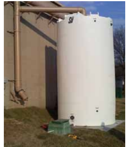
Figure 8. 6,000 gallon cistern (Papillion, Neb.)
