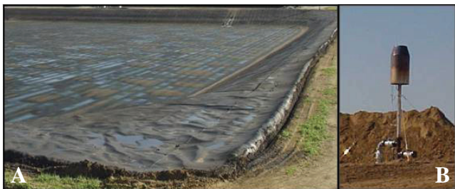
Figure 1. A) Covered anaerobic lagoon. B) Biogas flare
