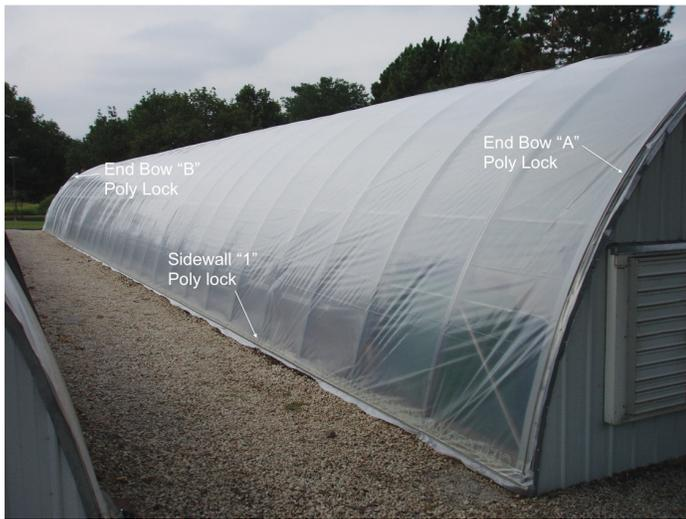
**Figure 18.** Locations of end bow and sidewall poly-locks.
