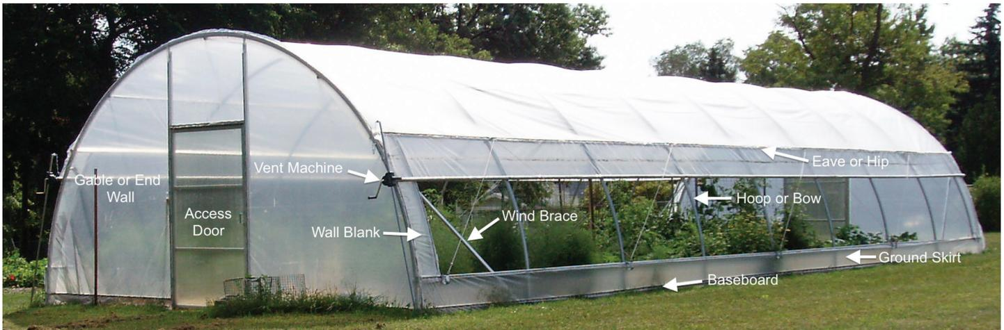
**Figure 1.** Common high tunnel terminology.
