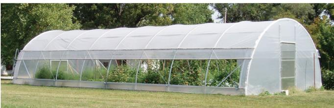
**Figure 5.** Roll-up sidewall components provide options for improved interior temperature management. Note overlapping wall blanks at both ends of the roll-up wall to prevent cold air infiltration.
