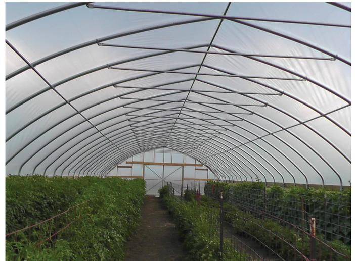
**Figure 11.** Cross bracing was installed in the peak of this high tunnel to stabilize the structure during high winds, heavy rains, and snowfall.
