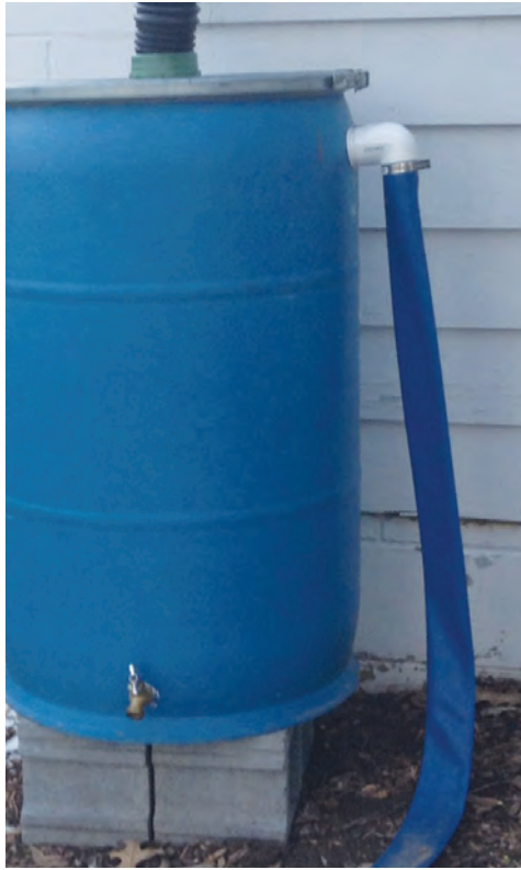
Figure 5. Flexible hose overflow option
