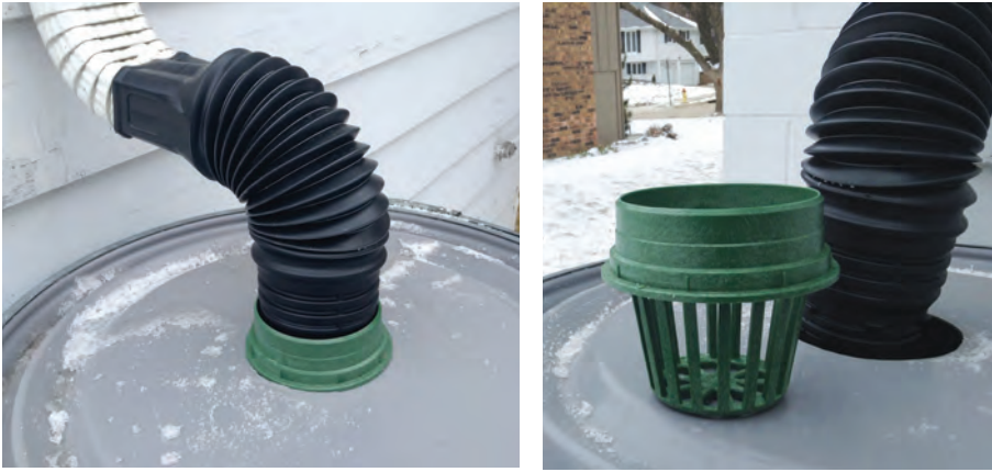
Figure 7. On left, flexible downspout adapter fitted into a 4-inch atrium grate. Atrium grate shown separately on the right. Screen can be fastened around the grate, but if the downspout adapter fits snugly into the grate opening, it isn't necessary. Be sure to clean the screen and grate frequently.
